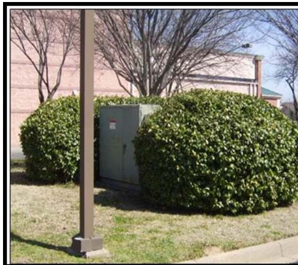
Figure 15.3-21. Ground-level Utilities Screening
